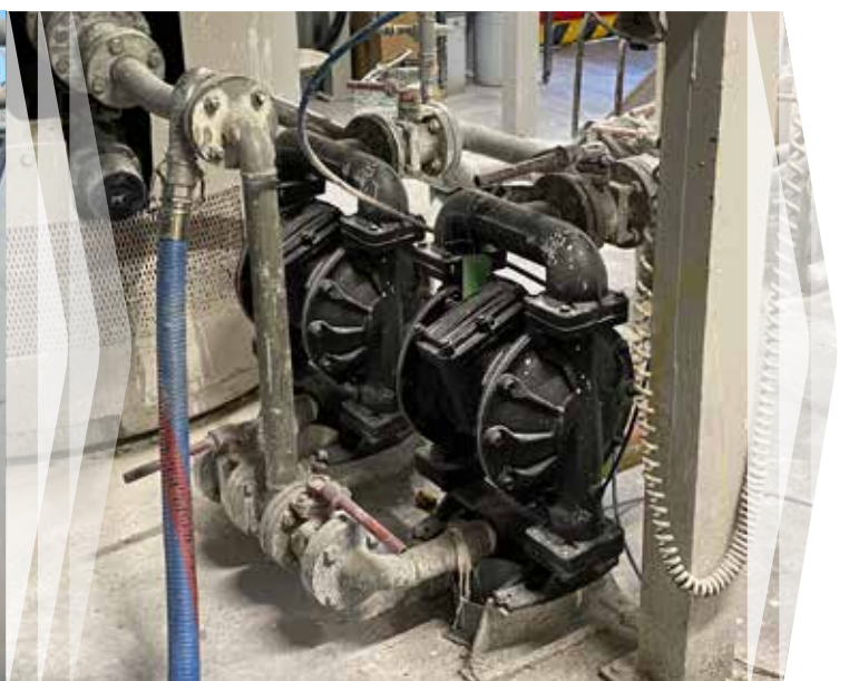
High fluid viscosity reduces pump delivery.
